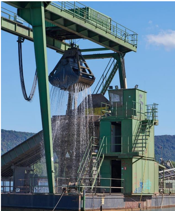
WET CUT: The gravel is dredged from a depth of more than 20 m using a floating-grab excavator.
