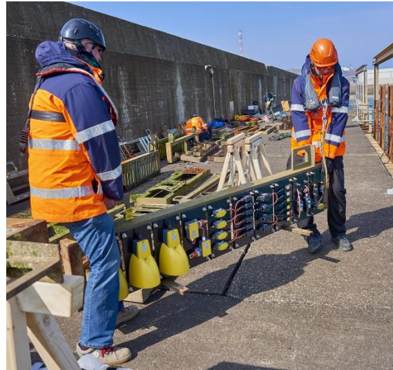
02 Parallel to the laboratory tests, the switching devices are also tested in real-life conditions – here at an outdoor test centre on the island of Helgoland
